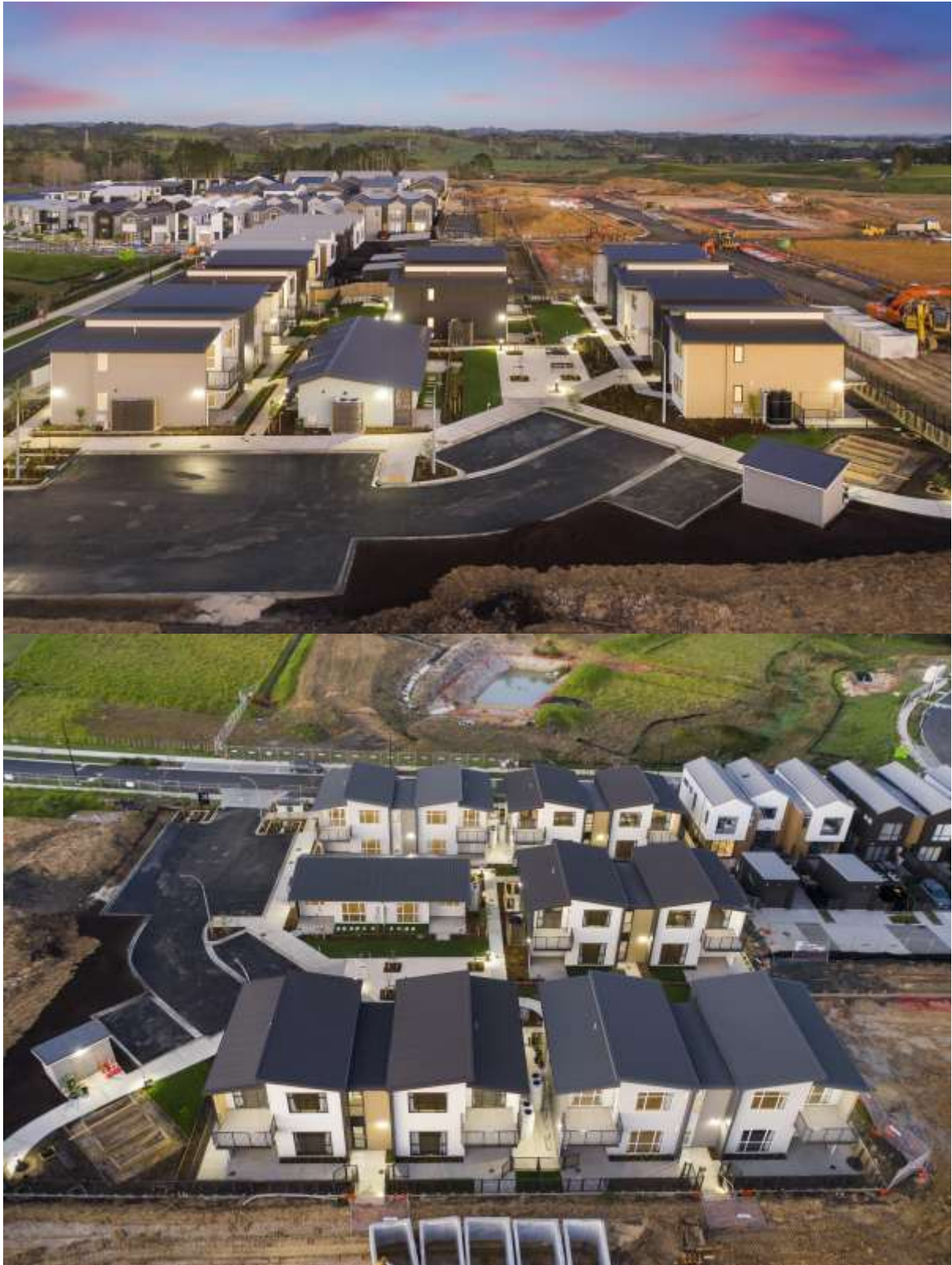
Photos of Te Manaaki Tāngata, The Salvation Army's 22-home development at Westgate, Auckland. These are part of the 118 new social housing units financed by The Salvation Army Community Bond.
